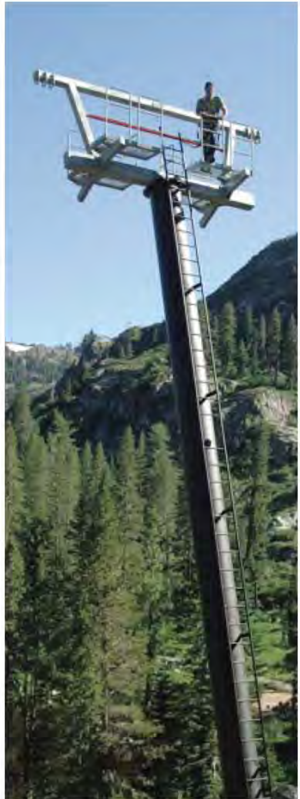
Caldwell says you design the towers for the wind load on the cables that run between them, not for the people on the chairlift. The towers are also pitched on the mountain at various degrees of lean. Caldwell welded these towers in his garage, which also houses his snowcat (shown at left).
