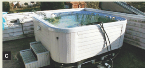
Fig. A: Collector box with black hose coiled inside. Fig. B: Intake and outlet hoses dangle in the tub. Fig. C: Solar-powered pump sits under the tub.
